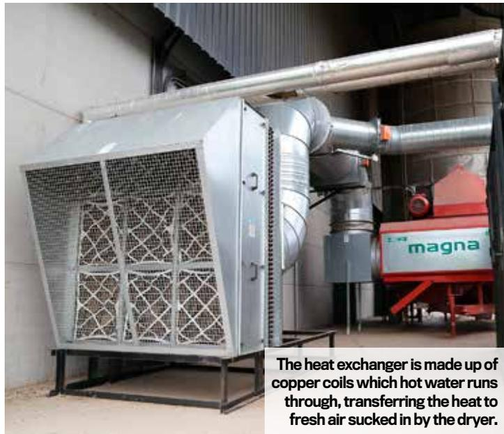
The heat exchanger is made up of copper coils which hot water runs through, transferring the heat to fresh air sucked in by the dryer.
