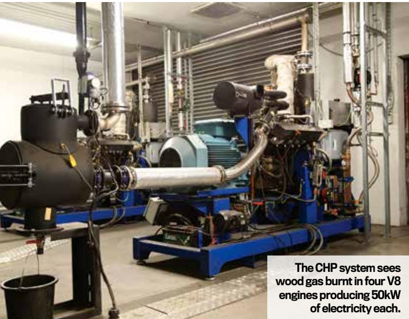
The CHP system sees wood gas burnt in four V8 engines producing 50kW of electricity each.
