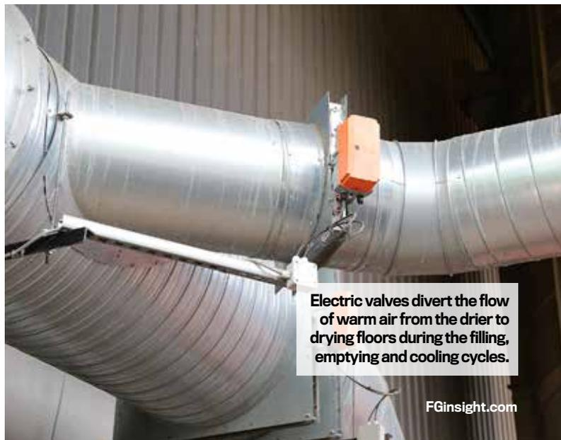
Electric valves divert the flow of warm air from the drier to drying floors during the filling, emptying and cooling cycles.
